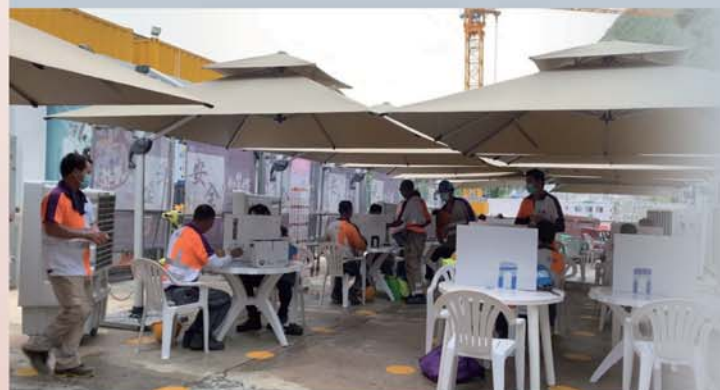
承建商於工地設立指定用餐區，每張餐枱相隔1.5米距離及限坐2人 Provision of designated dining area inside construction site with tables placed at least 1.5 meters apart from each other and a cap of 2 persons at each table
